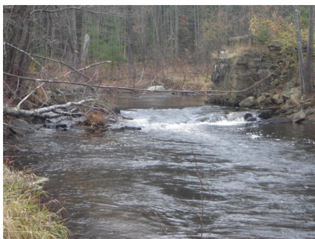
Photograph 7. Remainder of North Waterford Dam, 2011 (J. Pellerin).
